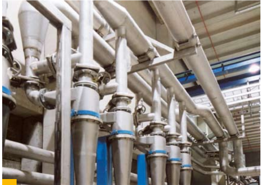
Fig. 9: Installed duplex pipeline
