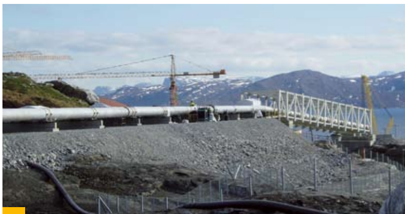
Fig. 32: Duplex pipeline after laying
