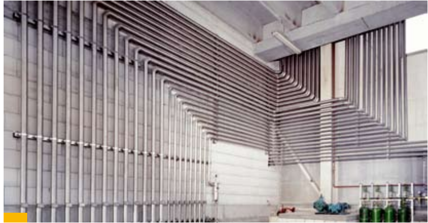
Piggable pipes and elbows are used in many industrial branches
