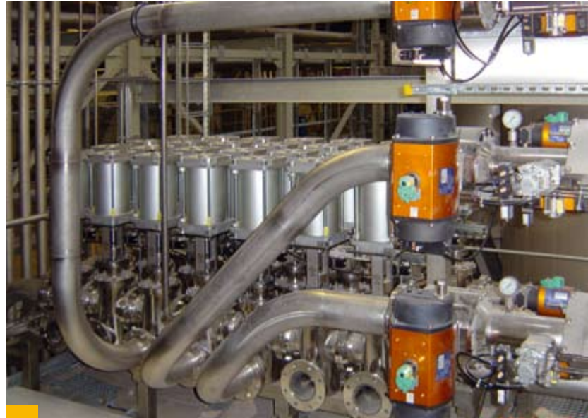
Bent piggable pipes from BUTTING
