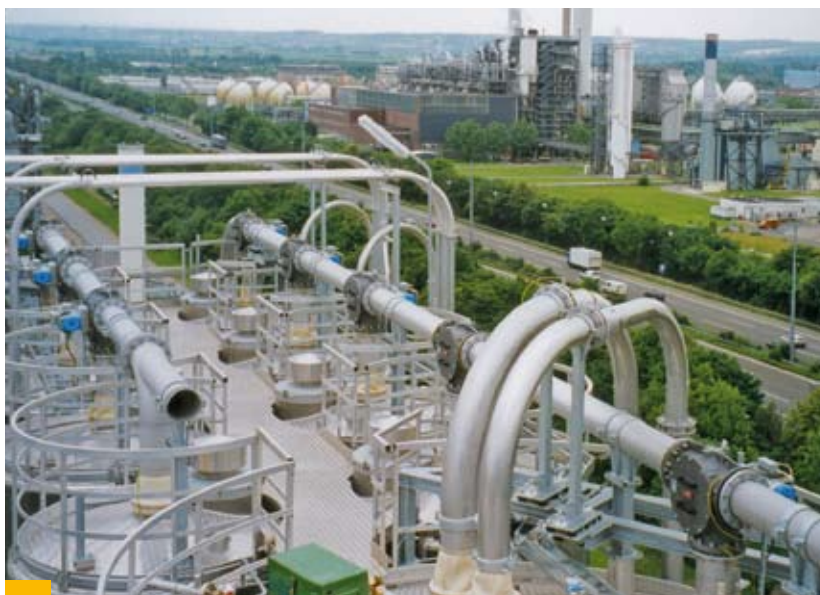
III. 11: Installation of special alloy products at a chemical plant
