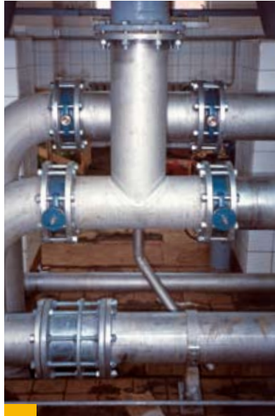
BUTTING makes extensive use of prefabrication to reduce costs
