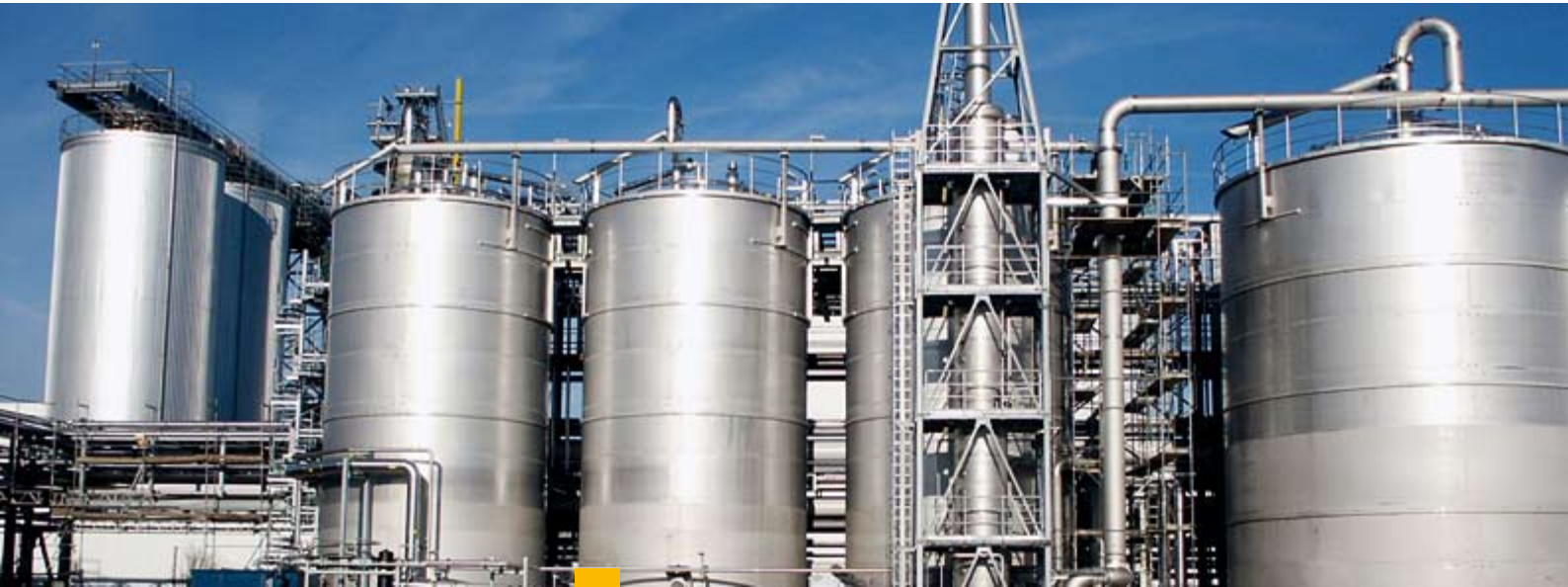
Prefabrication and assembly of pipelines and vessels by BUTTING Anlagenbau
