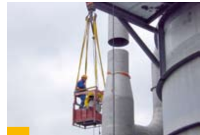
Installation of pipes up to 60 metres above the ground
